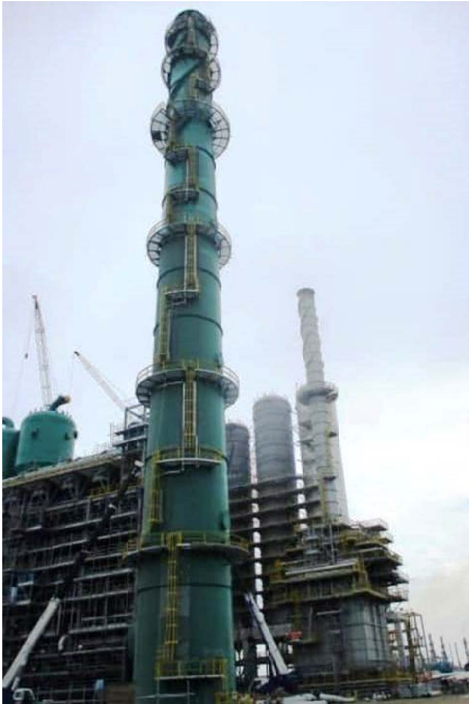
RDMP CO BOILER BYPASS STACK AT SITE (7800 ID x 89000 H ) 940 ton WITH REFRACTORY 175 MMt
